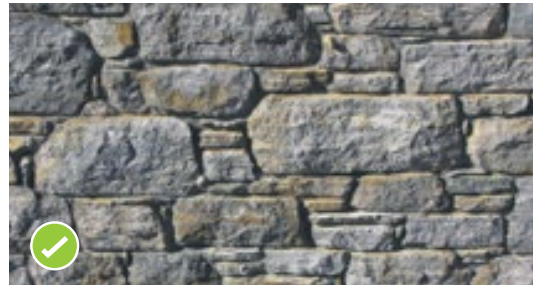
Figure 11 Acceptable stone work – joints are of an even size. Vertical joints are less than 300 mm high, and stones are regularly crossed to form good bonding. Source: NZSMA
