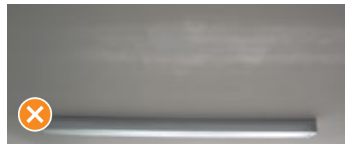
Figure 22 Sheen banding on a finished ceiling that is clearly visible from normal viewing position under non-critical lighting conditions. Source: Winstone Wallboards
